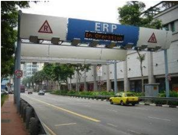
Abb. 17: ERP Gantry in Singapur
